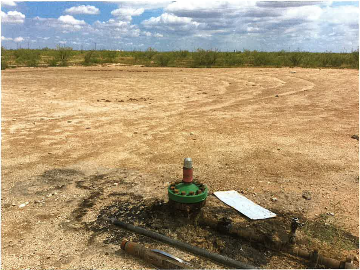
North Cowden Unit Well drilled during the Nixon years. Well is on a slope that drains into a playa lake. No vegetation to hold the rainfall causes the salts and other bad stuff to run into the playa. Under the proposed rules, this pit would be exempt from any regulation.
